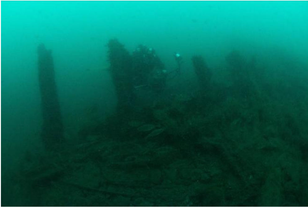
Figure 13: Framing of the vessel visible in the mid ships area behind the boilers
